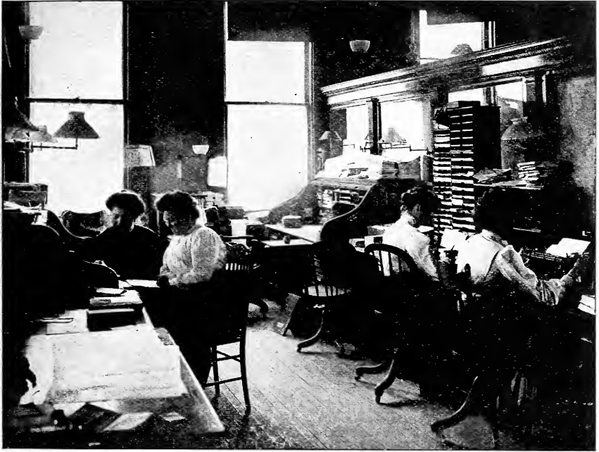
ONE OF SEVERAL CORRESPONDENCE ROOMS.
